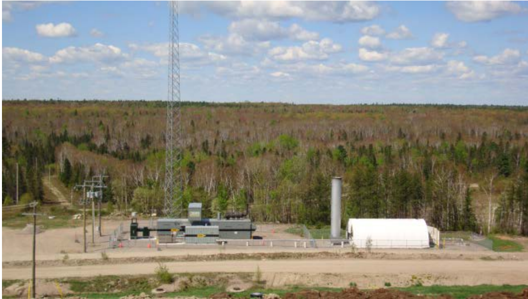
Figure 5: Landfill Gas Utilization to Electricity Facility and Landfill Gas Flaring Station located at the City’s Merrick Landfill Site
