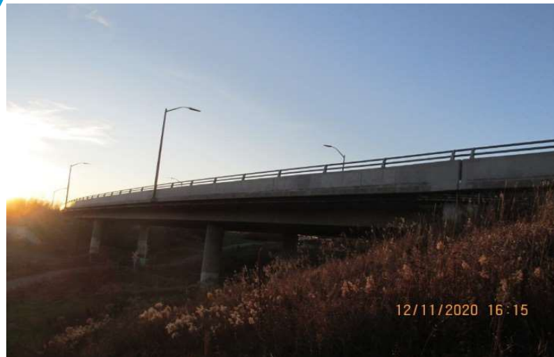
Trout Lake Overpass – Fair Condition
