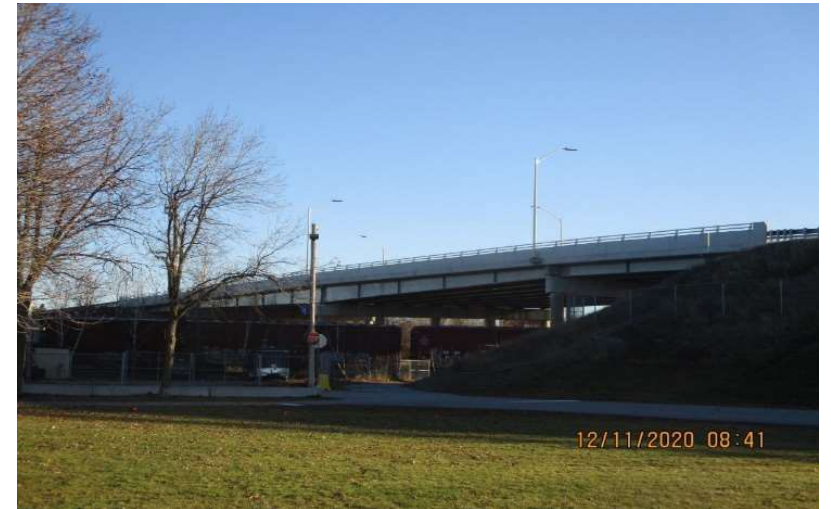
Very Good Condition – Lakeshore Overpass
