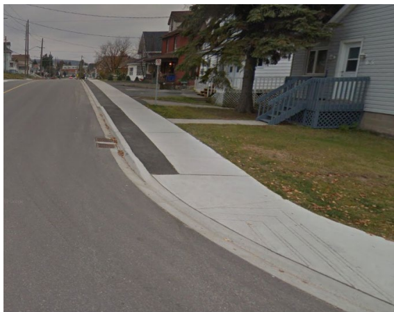
Sidewalk in good condition
