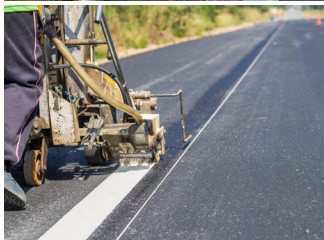
Enhanced Pavement Markings
