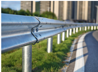
Guide Rail Upgrades
