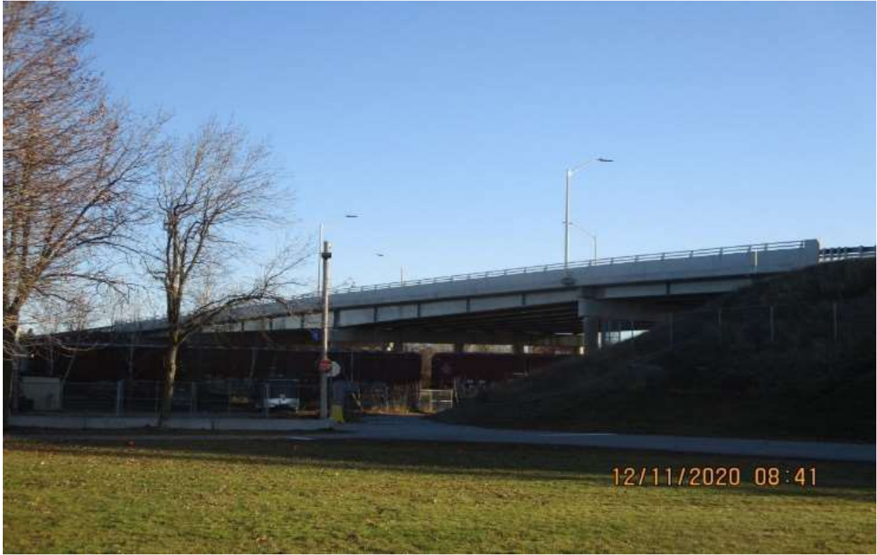
Very Good Condition – Lakeshore Overpass
