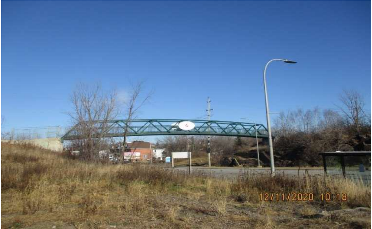
Kinsmen Pedestrian Overhead – Fair Condition
