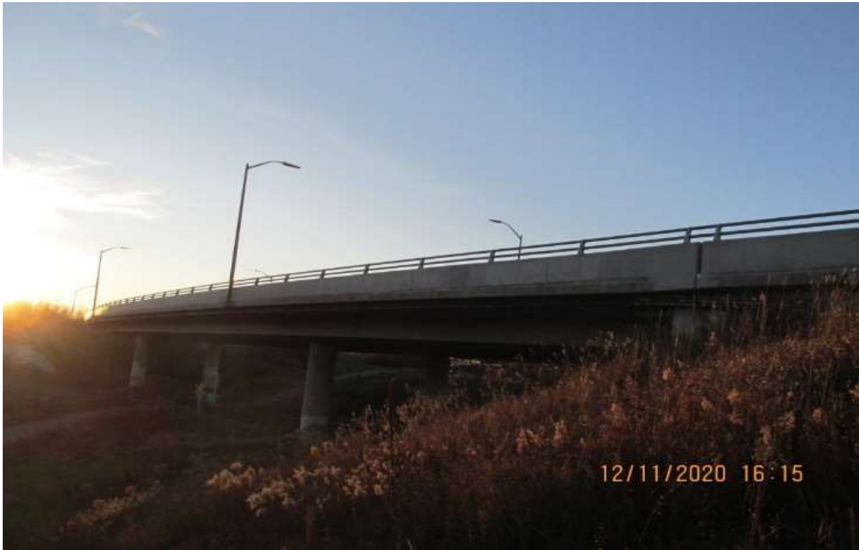
Trout Lake Overpass – Fair Condition
