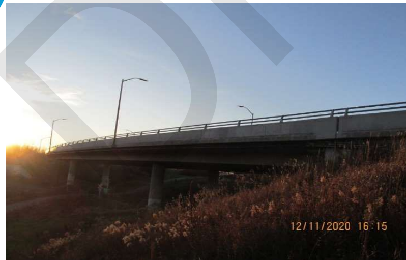
Trout Lake Overpass – Fair Condition
