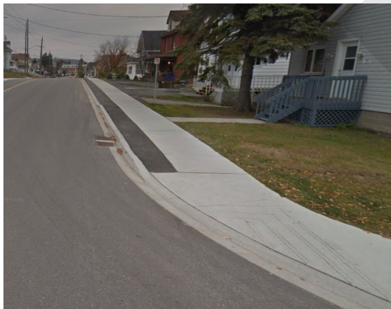
Sidewalk in good condition
