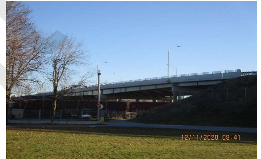
Very Good Condition – Lakeshore Overpass
